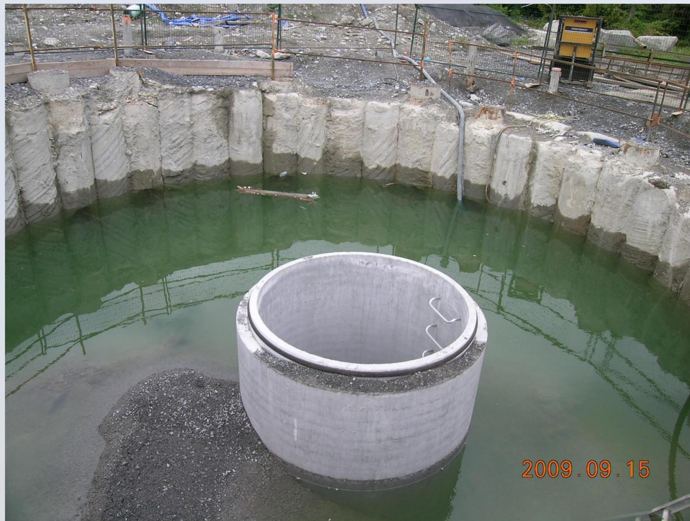
Groundwater infiltration in rock excavation /
